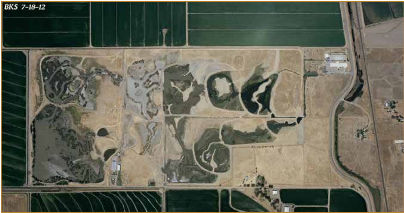
FIGURE 7 The Conservancy's flagship marsh complex. Shown by aerial photography in 2012, the Conservancy's Betts, Kismat and Silva preserves (collectively known as BKS tracts) are a reliable refuge for giant garter snakes. Ponds M and N in the center-left portion of the photo can be seen completely de-watered as they await channel renovation.
