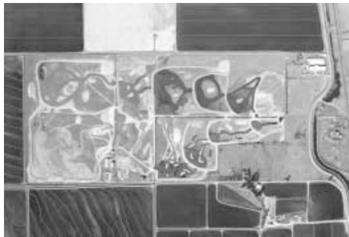
Betts-Kismat-Silva Restoration and Enhancement construction project, December 2001. Aerial photo showing restoration and enhancement construction completed. Vegetation planting beginning. Note sinuous marsh areas and basking islands for the benefit of the giant garter snake. Photo: CalAero for The Natomas Basin Conservancy.
